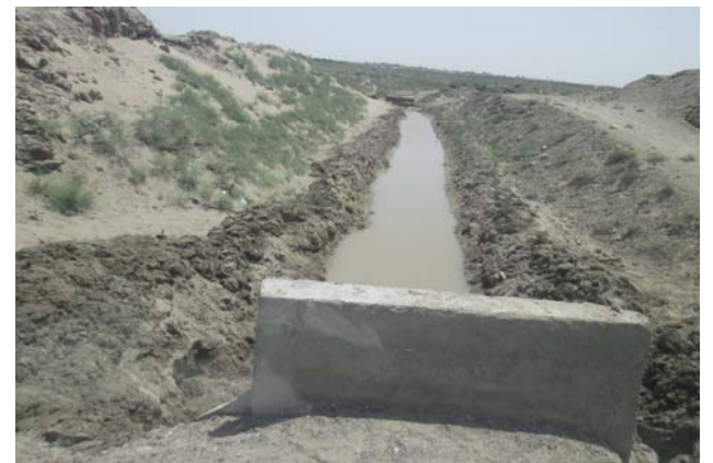
Figure 15; Sub-canal of Haji Rahatullah, Haji Abdul Rahman Ragi takes water from Lashkari Canal for irrigation of 216 hectare of area
