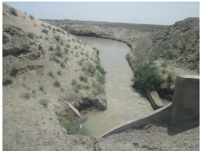
Figure 11; Sub-canal of Haji Ali Khan, Bainaz initiates from Lashkari Canal irrigates about 140 hectare land
