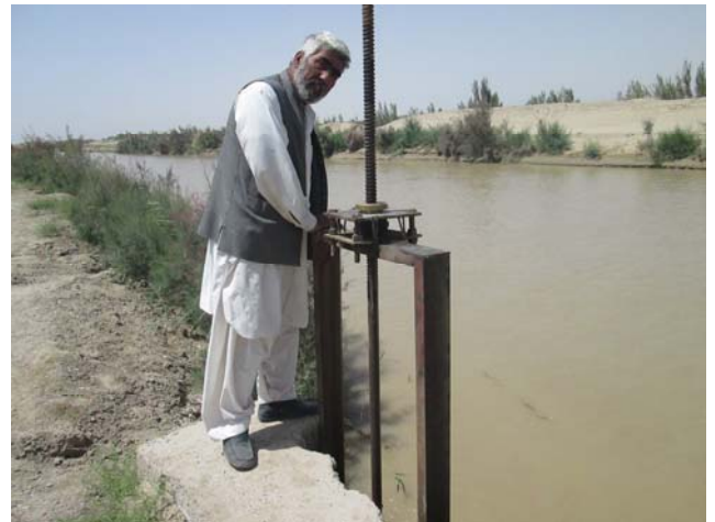
Figure 13; A control installed over Lashkari Canal for controlling flow of water to sub-canal; however the proprietor of jui welded the gate open to avoid its closing by mirabs to get more water than supposed to
