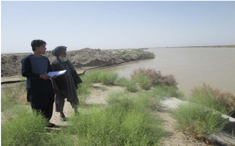
Figure 3; Initiation of Lashkari Canal (Left Side) which diverts water from Helmand river (Right Side)
