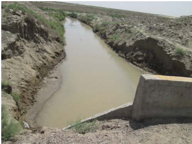
Figure 14; Sub-canal of Haji Alim, Shuraw initiates from Lashkari Canal and irrigates 357 hectare land
