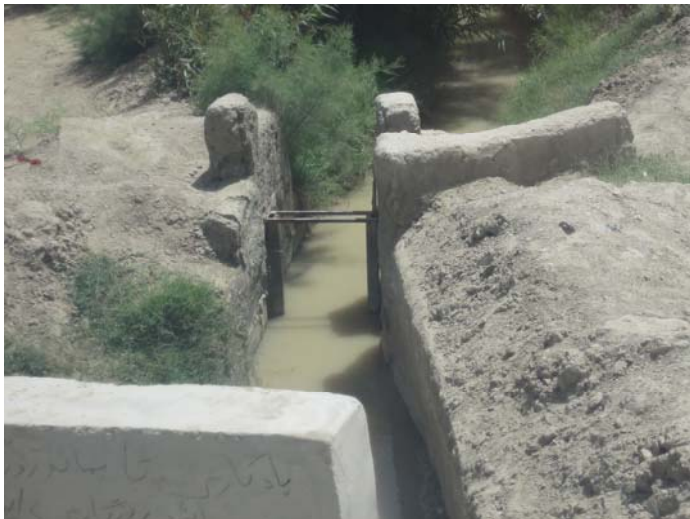
Figure 24; Sub-canal of Kalokhak from main canal If Lashkari irrigates 131 hectare area
