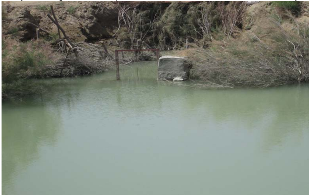
Figure 9; Illegal gate built on Lashkari Canal's escape way
