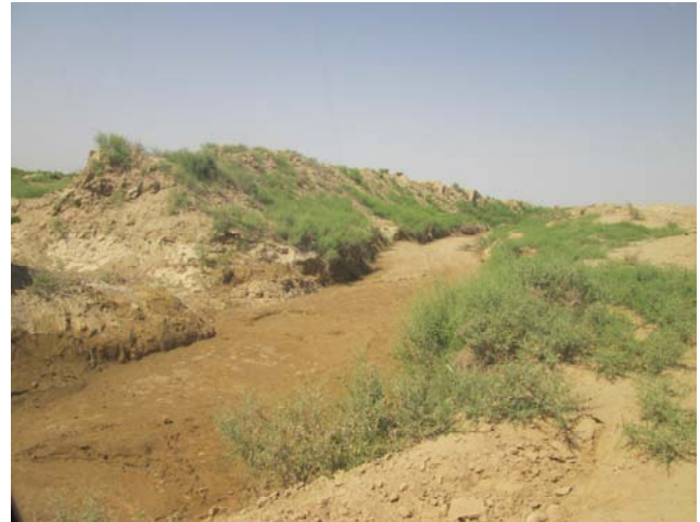
Figure 39; Sub-canal of Haji Halim Walidi Noorullah initiates from Lashkari Canal irrigates 240 hectare land
