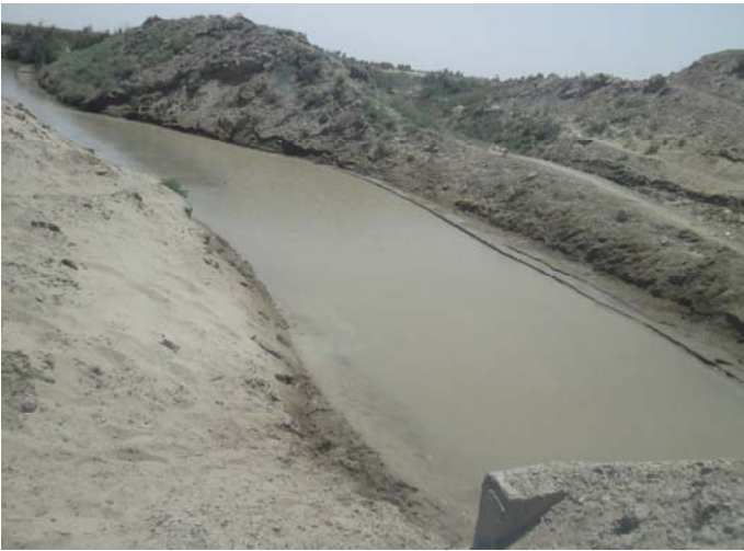
Figure 12; Jui Araf, Dasht Khawabga initiates from Lashkari Canal and irrigates 100 hectare land
