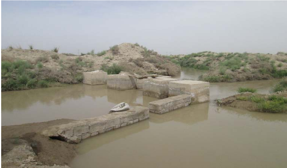
Figure 6; Distribution of water in Kang District. Unlike Zaranj, people do not have control gates for controlling amount of water, and they use such structures from clay or concrete for this purpose
