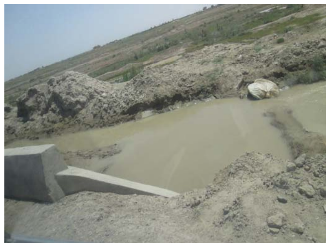
Figure 19; Sub-Canal of 9 Haji Zaher, Sardasht initiates from Lashkari Canal irrigates 402 land
